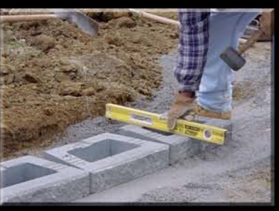
8. When 2 to 4 courses of block have been placed in your wall and properly aligned you will fill the core of the blocks and two feet behind the wall with #67 crushed stone.
