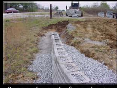
9. Sweep the rock from the top courses of block. Place additional courses of block on the wall repeating the construction process until the desired wall height is achieved.
