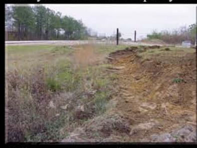
1. Dig a two foot wide foundation trench 6 to 12 inches deep removing soft surface top soils.
