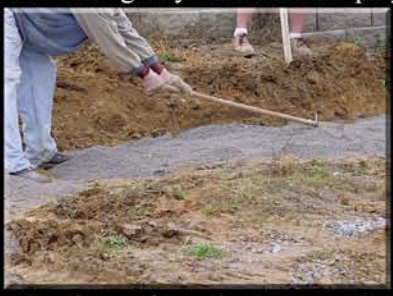
2. Rock foundation & leveling pad. Crushed rock is placed 2 to 4 inches deep in trench and leveled.
