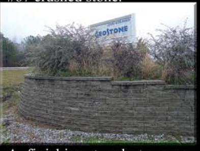
12. A finishing touch to your wall is a cap block that can be applied with outdoor construction glue.
