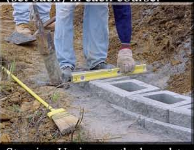
11. Stepping Up is a method used to follow a slope up hill. The base course runs into the ground as shown while the course above continues on. Make sure to level each footing block in the step up procedure.
