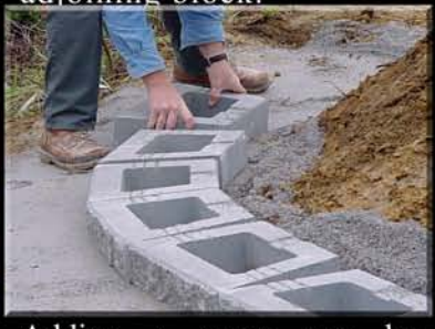
10. Adding a curve can be achieved easily due to the shape of the block and its not being hindered by lips or pins.
