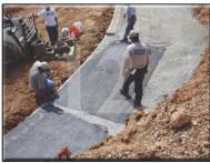
Next lay out the geogrids. Their length will depend on the wall height. Rule of thumb is no less than 75% of wall height (no shorter than 4') and no less frequent than every 2 vertical feet.
