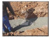
The footing depth will vary based on the the height of the wall. Rule of thumb is 1 inch of embedded block per vertical foot of wall height is required. Place four to six inches of crushed rock (#78 or #8910) in the footing and level for the wall foundation.
