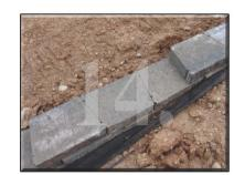
This process is repeated until the desired wall height is reached. The final course is the cap block glued down with outdoor construction adhesive.
