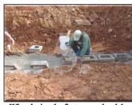
When laying the first course, level the block front to back and side to side with a two foot carpenter's level. It is very important that the first course be placed on a compacted footing and leveled before preceding.
