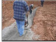
As preparation of the footing continues, remove all large rocks and use a vibrating plate tamp to achieve proper compaction. Get footing as smooth, level, and compacted as possible.
