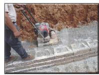
Compacting the backfill is very important. This provides additional resistance to pressures exerted on the wall and prevents settlement. Repeat this process after each backfill.
