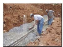
Sweep all rock and gravel from the tops of the blocks before laying down next course or geogrids. Any variance in height caused by rocks between courses will cause unsightly gaps. Backfill area should encompass entire proposed grid length area.
