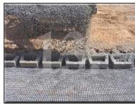
After laying out the grids, place another course of block down on top of the grids, align, then core fill and backfill. It is important that the grids be stretched tight prior to placing rock fill.
