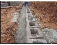
Align and batter each course prior to core filling with rock. Batter means setting each course back 1/4 - 1/2 inch behind the course below as seen in the picture above. On straight walls, use a string line. In curves, visually align the wall to achieve the desired appearance.
