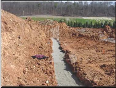
Begin by digging a two foot wide trench. Excavate all loose soils and native rock until hard original ground is reached. The footing will be supporting the entire weight of the wall.
