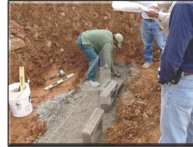
Run a string line for straight walls. This will help in the alignment of the first course. Use a cement trowel to smooth out base prior to setting first block.
