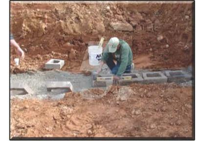
When laying the first course, level the block front to back and side to side with a two foot carpenter's level. It is very important that the first course be placed on a compacted footing and leveled before preceding.
