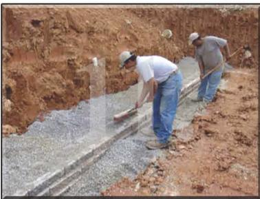
Sweep all rock and gravel from the tops of the blocks before laying down next course or geogrids. Any variance in height caused by rocks between courses will cause unsightly gaps. Backfill area should encompass entire proposed grid length area.
