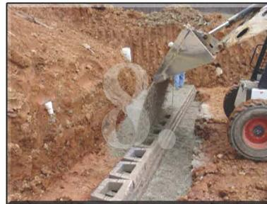
It is recommended that the cores of the block be filled with a #67 or #78 stone no less frequently than every three courses. This same stone is recommended for the backfill as well.
