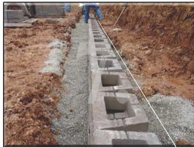
Align and batter each course prior to core filling with rock. Batter means setting each course back 1/4 - 1/2 inch behind the course below as seen in the picture above. On straight walls, use a string line. In curves, visually align the wall to achieve the desired appearance.
