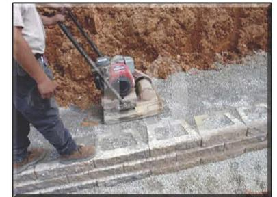
Compacting the backfill is very important. This provides additional resistance to pressures exerted on the wall and prevents settlement. Repeat this process after each backfill.
