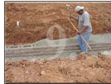
After core filling the block, use a rod to drive down into the cores to assure a thorough core fill. Backfill should be level to top course of block.
