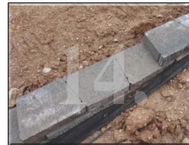
This process is repeated until the desired wall height is reached. The final course is the cap block glued down with outdoor construction adhesive.
