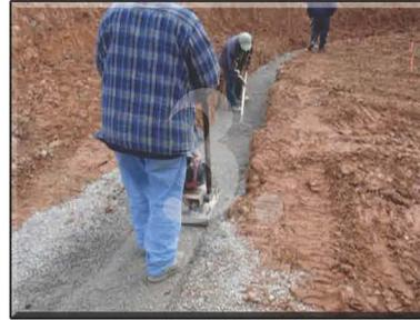
As preparation of the footing continues, remove all large rocks and use a vibrating plate tamp to achieve proper compaction. Get footing as smooth, level, and compacted as possible.
